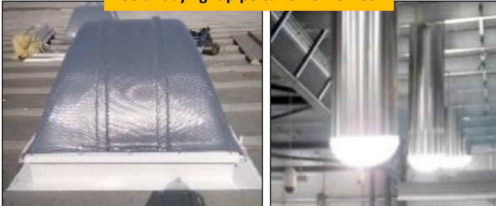
Solar day light pipe & Dome 46 Nos
